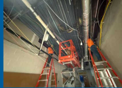
Structural Steel Installation
